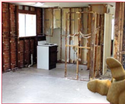
▼ $10,000 damage, not covered by insurance.
