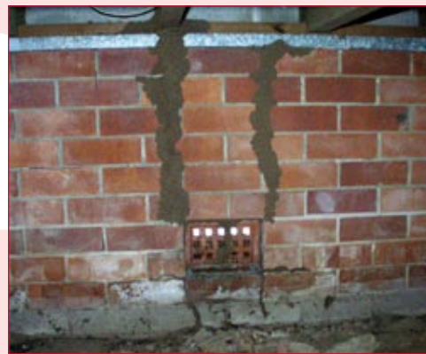
▼ Termites building mud tunnels up the brick wall and over ant capping.
